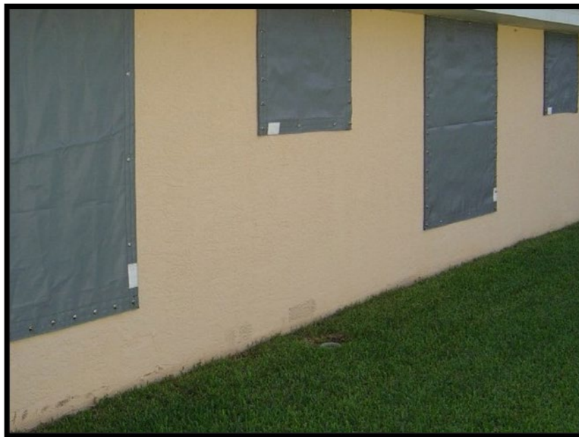
Figure 7 Example of attachable fabric hurricane wind screens (aka Storm Catcher Wind Screens) may be installed only after Collier County declares a local state of emergency for a potential hurricane event or other natural disaster and must be removed after the storm passes.
