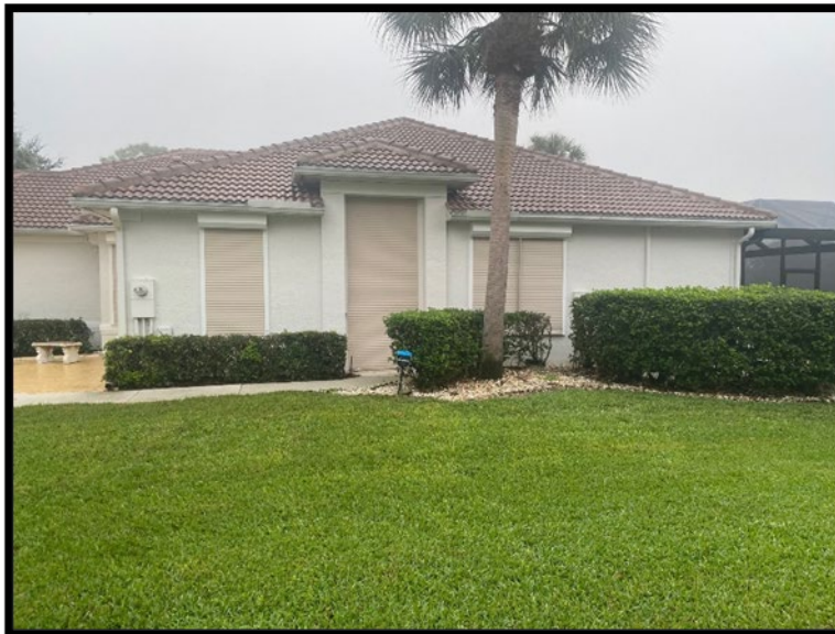
Figure 4 Example of roll down shutters with a compatible color that can remain rolled down during the hurricane season.
