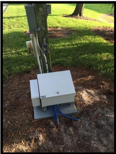
*Figure 3: Picture of electric compressor equipment that will provide air to the lake diffusers via air tubes. Lake diffusers (bubblers) will be located at the bottom of the lakes.*
