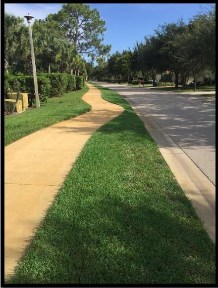
*Figure 1: Picture above depicts rust staining on sidewalk along Autumn Woods Blvd caused by iron in the lake irrigation water.*
