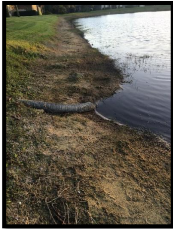
Figure 1: Picture to the left depicts a washout created by a flex pipe downspout.
