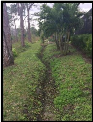
Figure 3: Ditch along Nature Preserve Ct that will be regraded and filled in partially to comply with slope standards.
