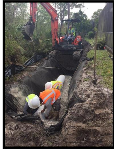
Figure 2: Picture to the right depicts the perforated pipe and rock trench for the exfiltration system behind some of the homes on Nature Preserve Ct.
